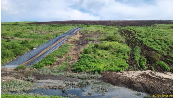
Erosion Along South Slope
