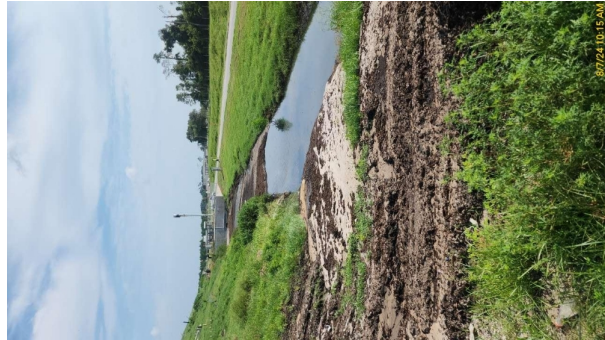
Erosion Along East Slope
